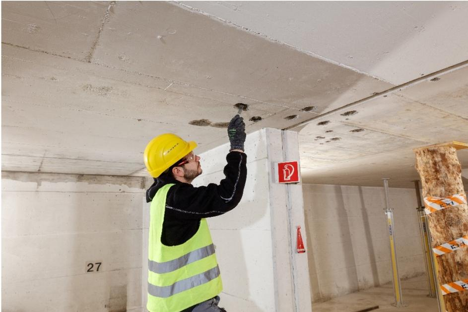
Fig. 29 Installtion of HZA-P anchor
