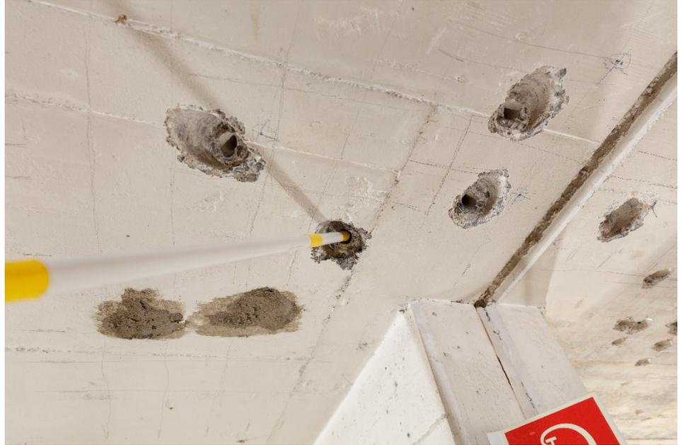
Fig. 28 Injection of mortar (End position)
