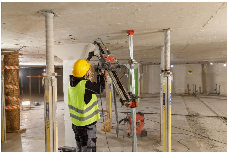
Fig. 21 Drilling with special drilling stand and hollow drill bit for automatic borehole cleaning
