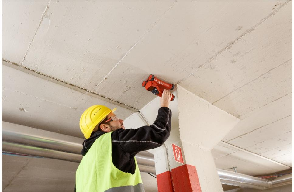
Fig. 20 Location of reinforcement with Ferroskan PS 200
