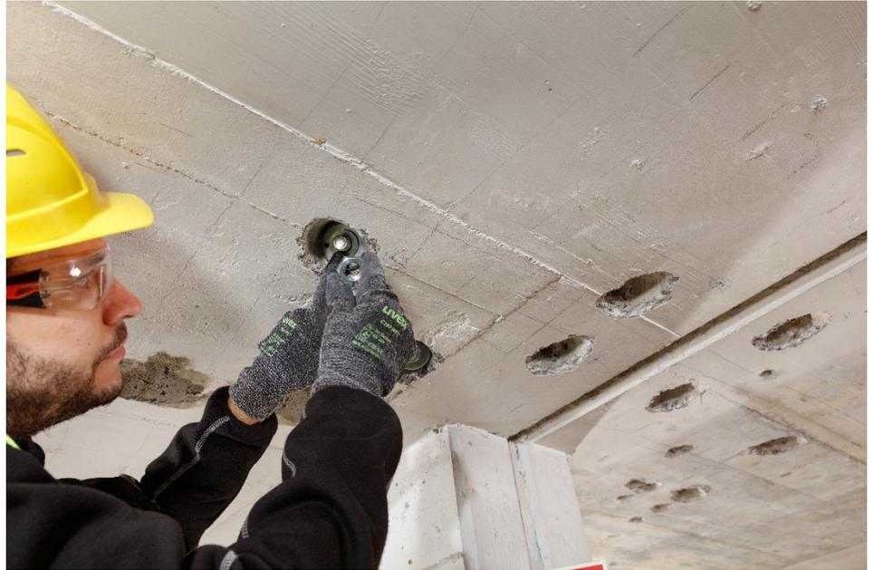
Fig. 30 Installation of anchor head
