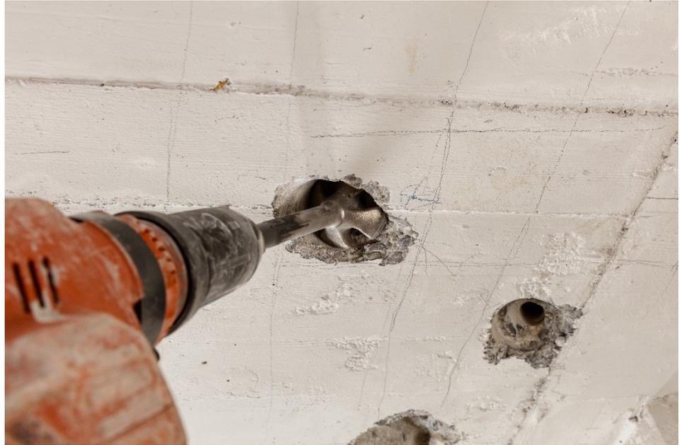
Fig. 23 Widenin of borehole with special srill bit TE-Y-GB
