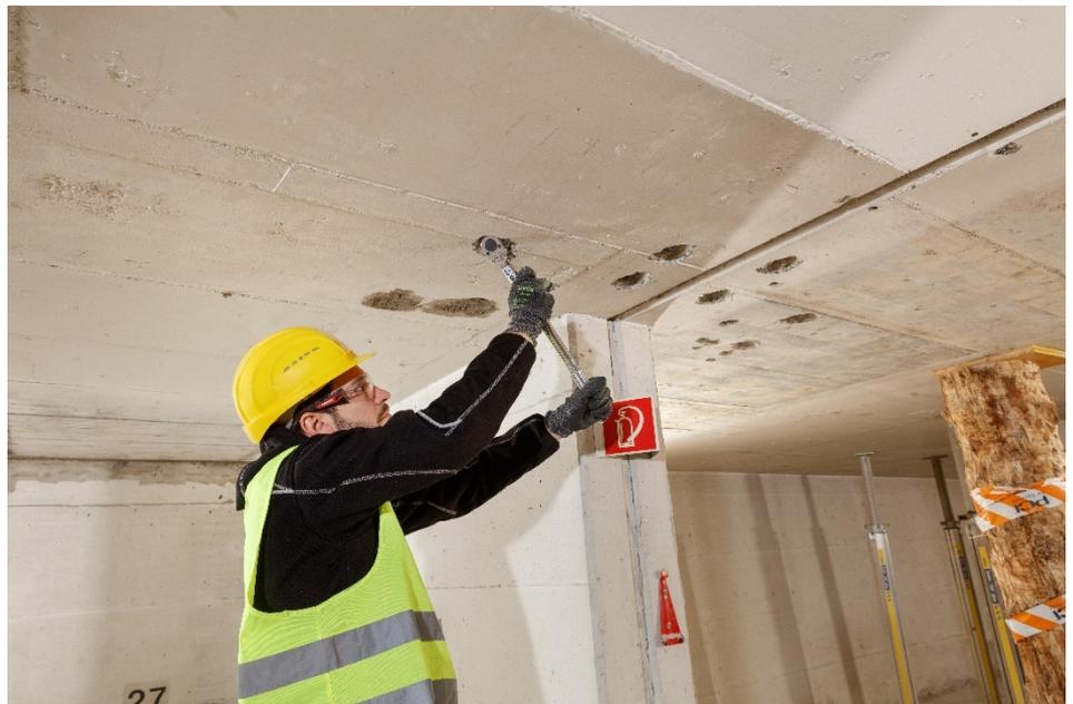
Fig. 31 Application of torque moment
